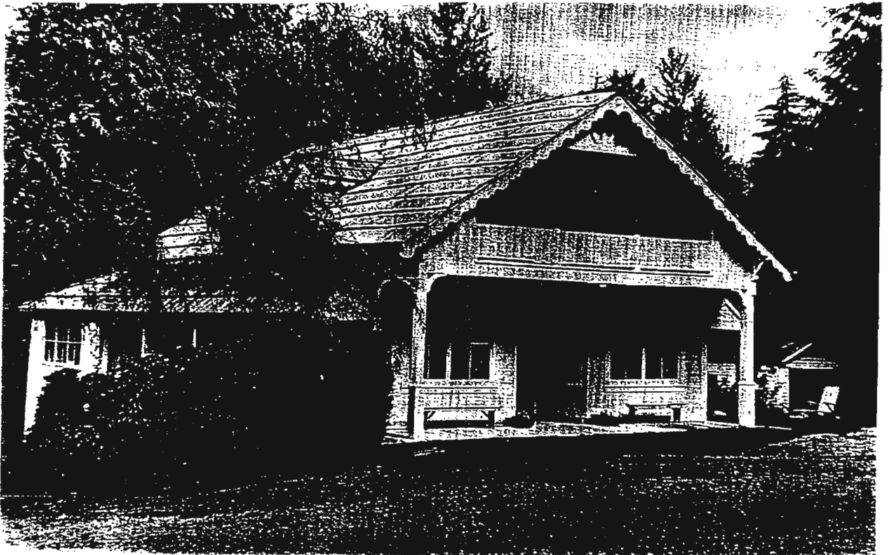
HM12 Poch's house built in 1923 with lumber from the Melmont schoolhouse. Photo: Caroline A. Gallacci, Office of Historic Preservation, Tacoma
